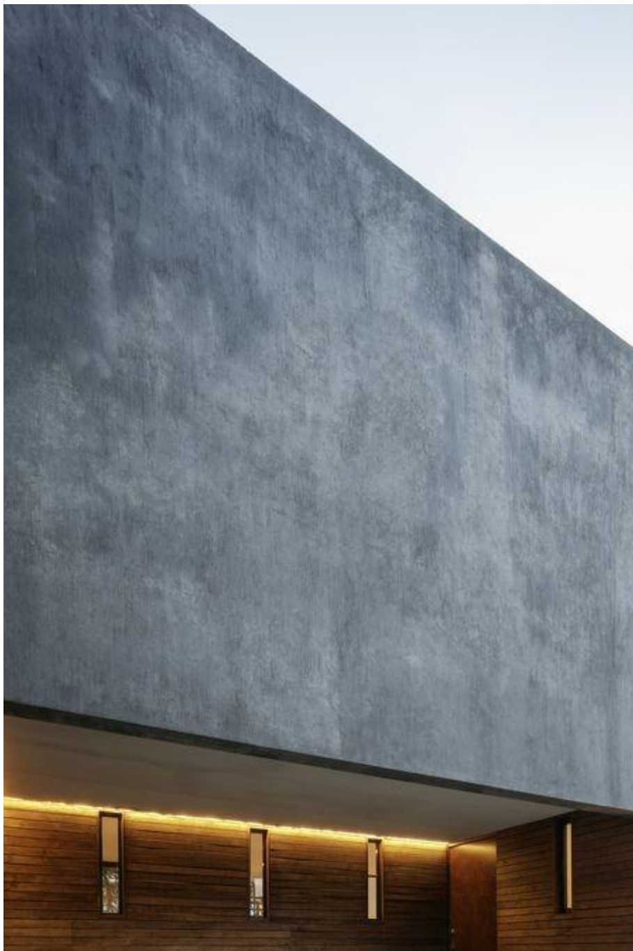
PC02 - PRECAST CONCRETE FACADE - MINERAL STAIN PAINT - DARK GREY COLOUR OR SIMILAR
