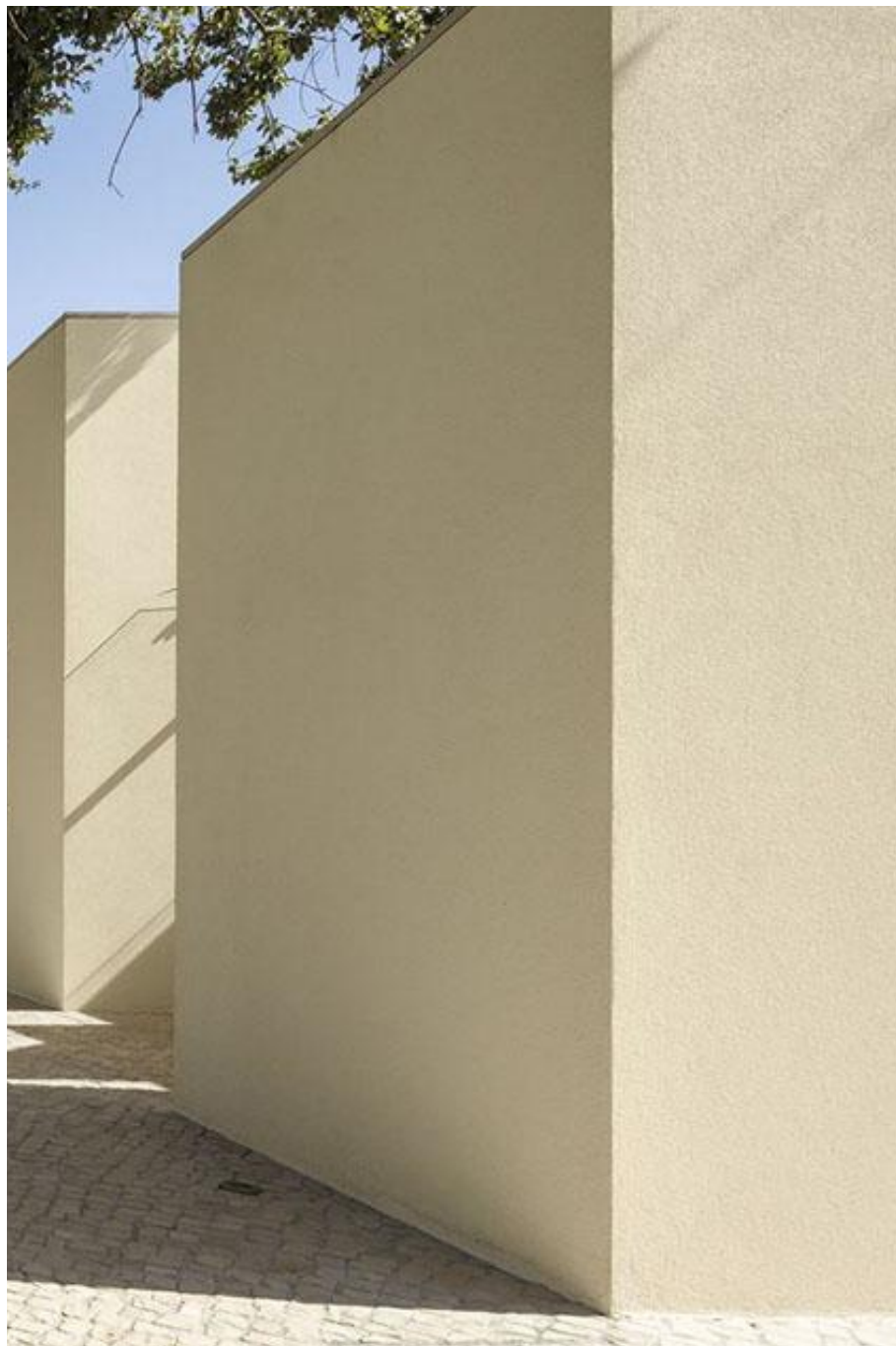
PC01 - PRECAST CONCRETE FACADE - MINERAL STAIN PAINT - SANDSTONE COLOUR OR SIMILAR (FOR PODIUM)
